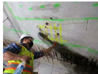
Half-cell testing for reinforcing steel corrosion
