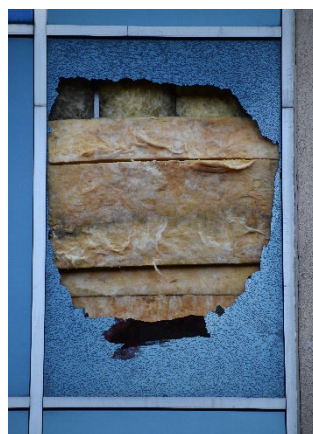
shattered spandrel glass within existing curtain wall system with exposed mineral wool
