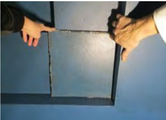
Using sample panles to verify paint color, glaze, and texture
