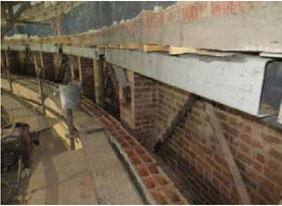
New structural support below plaster dome
