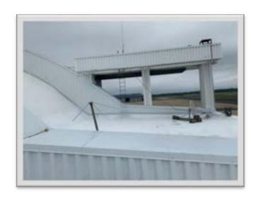
At Hangar 101 and 144, 100 percent of the existing roofs were replaced. At Hangar 109, the center section of the roof was previously replaced, so design included tie-in details between new and existing construction. All buildings remained fully occupied and functional for users during construction.
