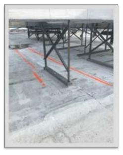
center paver area was installed to support the building research activities. Precast concrete paver walkways were installed to provide access to catwalks from the adjoining roofs. At the penthouse roof, structural steel elements set very close to the roof required coordination with roofing system manufacturer to obtain details that would perform as well as be covered by the required 20 year system warranty.
